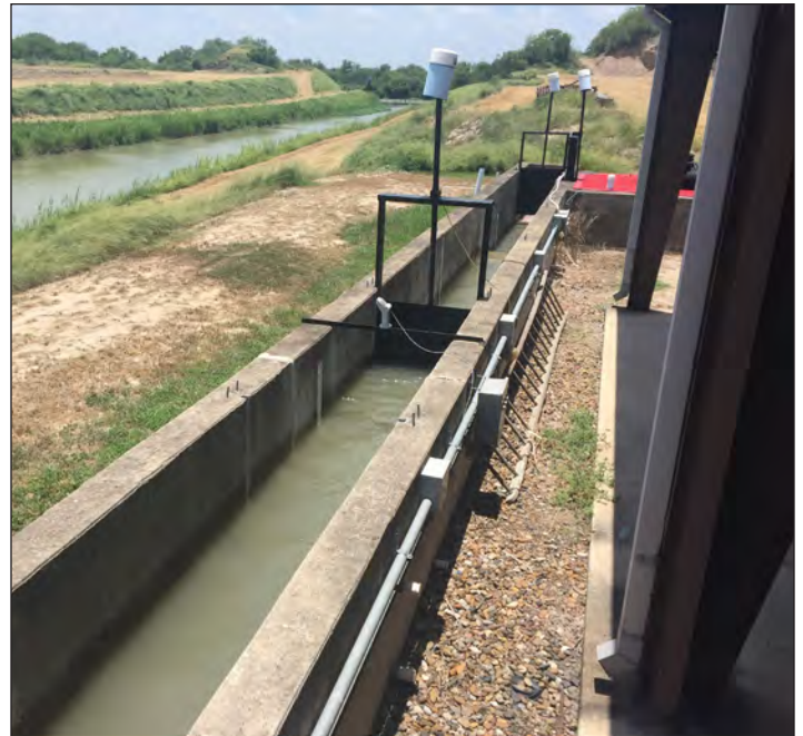
Water level sensor and automated gates in the demonstration channel at the Rio Grande Center for Ag Water Efficiency.
