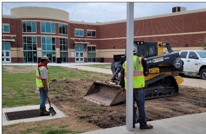
Removing the invasive grass and 2 inches of dirt. Photo by Jaime Flores.
